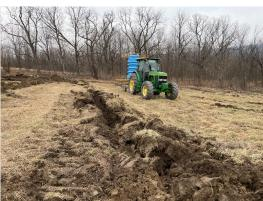
With the unseasonably mild weather, we're continuing our drainage tile project. The equipment in the pictures above place drainage pipes (called tiles) in the vineyard to remove excess water and help keep the vines' roots healthy.
